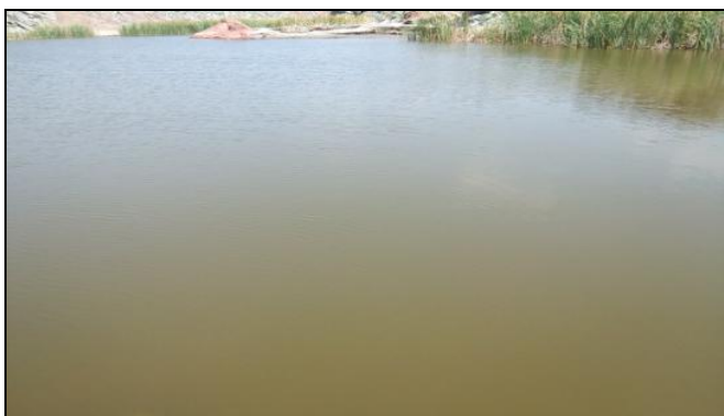
Fig 2: An overview of Nashpa dam
